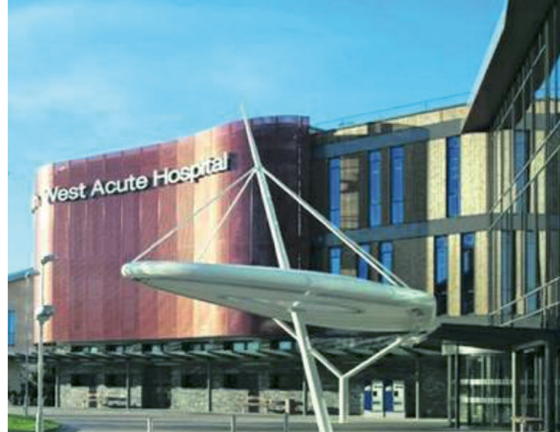
South West Acute Hospital, Enniskillen, Northern Ireland
