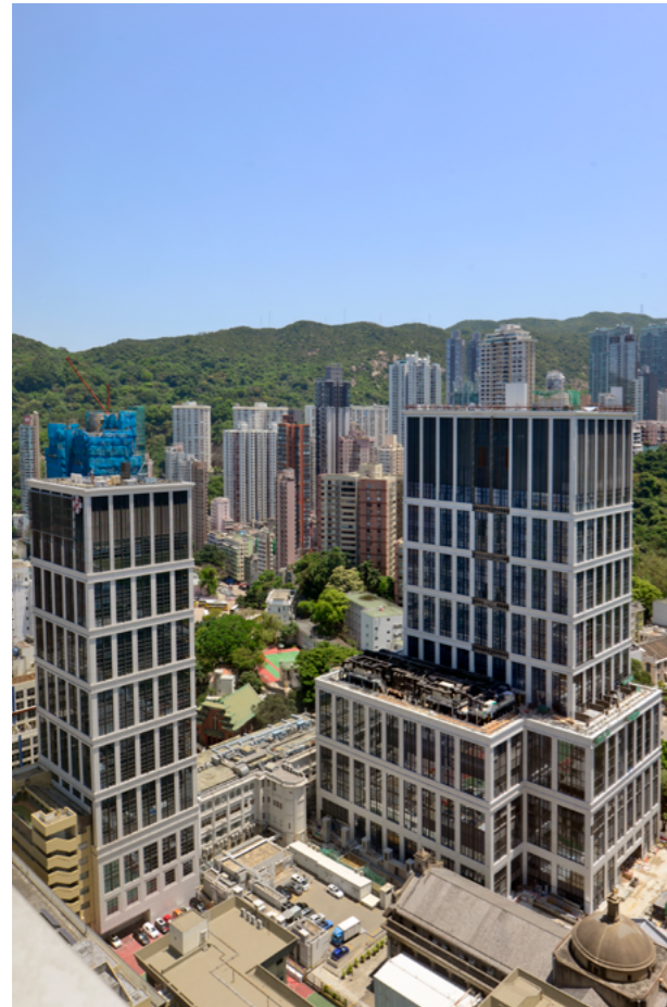
St. Paul's Hospital, the construction site abuts a historic chapel, three schools and a frequented hospital in full operation
